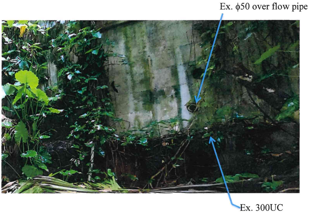
Photo 3: Photo showing the existing 300UC and \phi 50 over flow pipe
