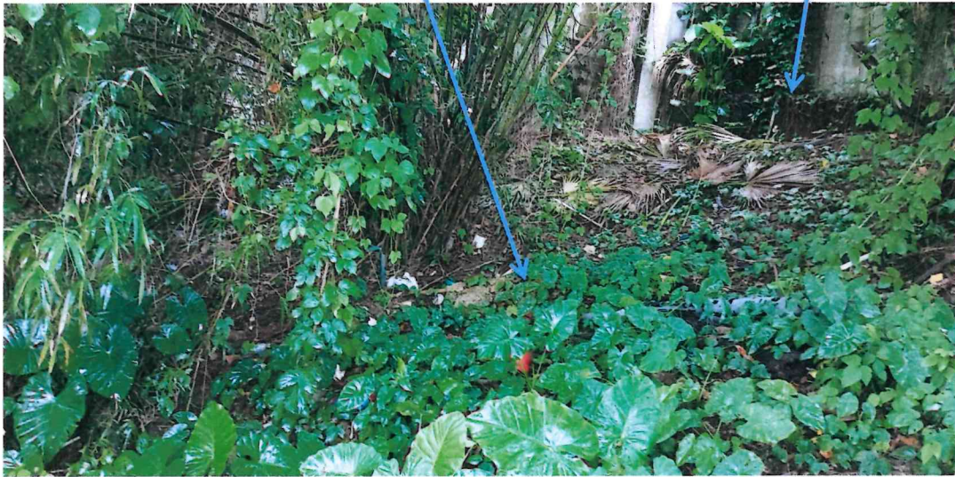
Photo 5: Photo showing the existing 300 stepped channel and catchpit
