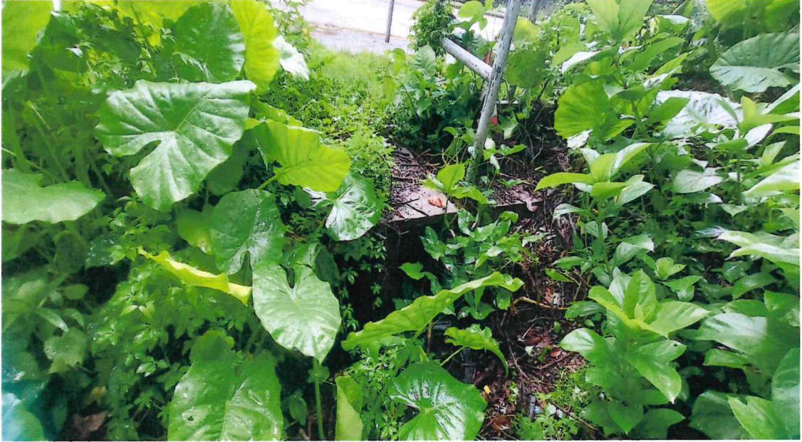
Photo 7: Photo showing the existing outlet
